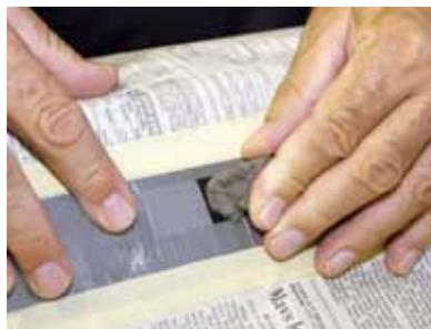
**8** Masking tape and newspaper was used to shield the remaining portions of the engine. Small quantities of cement were carefully packed into the opening. As the hole filled up, it became more difficult to force in the cement, but it must be completely filled. Any air pockets can collapse, compromising the cement's integrity.
